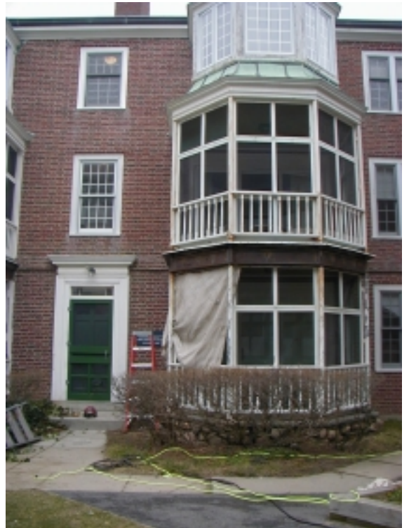
Porch structural repairs to the Brick Apartment Building.
